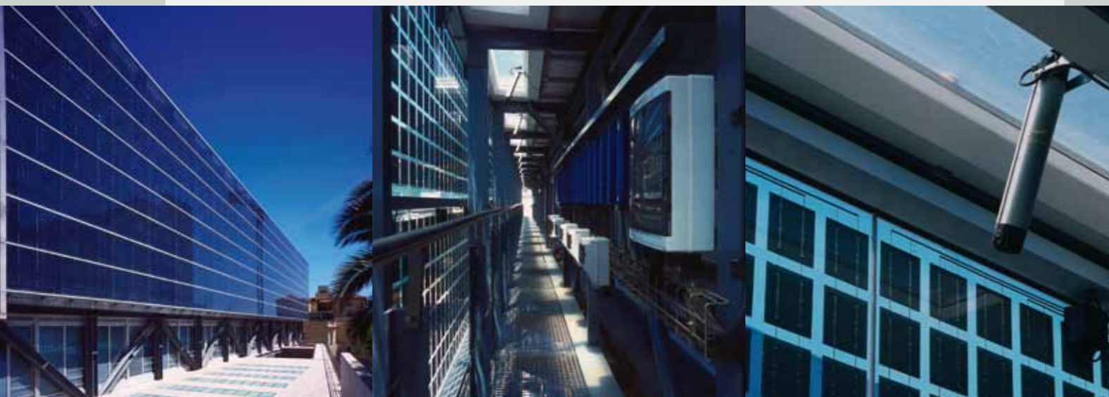
Curtain wall with photovoltaic panels - La Salle - Barcelona, Spain (Architect : Robert y Esteve Terradas Muntañola)
